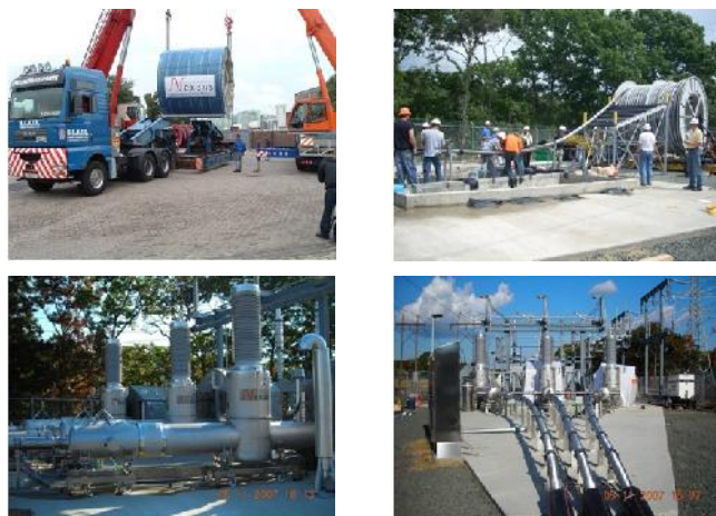
Cable successfully energized on April 22, 2008
