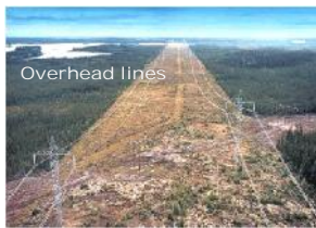
Nelson River DC line (Canada) 1600+1800 MVA (+2000 under construction)
